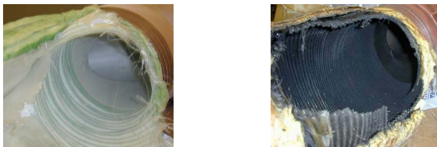
Figure 1. (left) Opened-up new ducting; (right) "in use" ducting [16].
